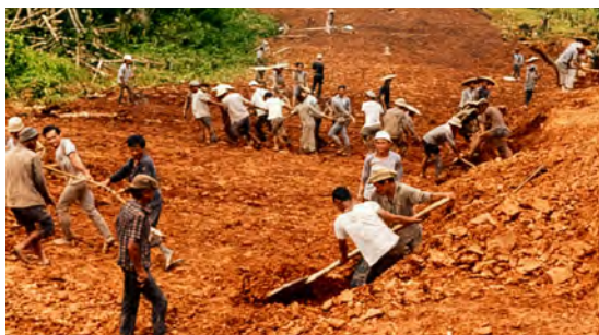
Working hard together with villagers in Long Jawi to build an airstrip, 1970.
